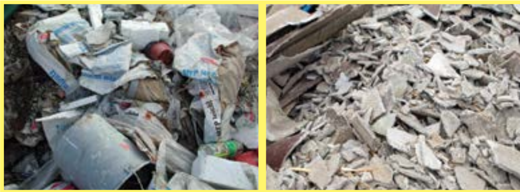
Figure 50: Construction site waste – Y46
