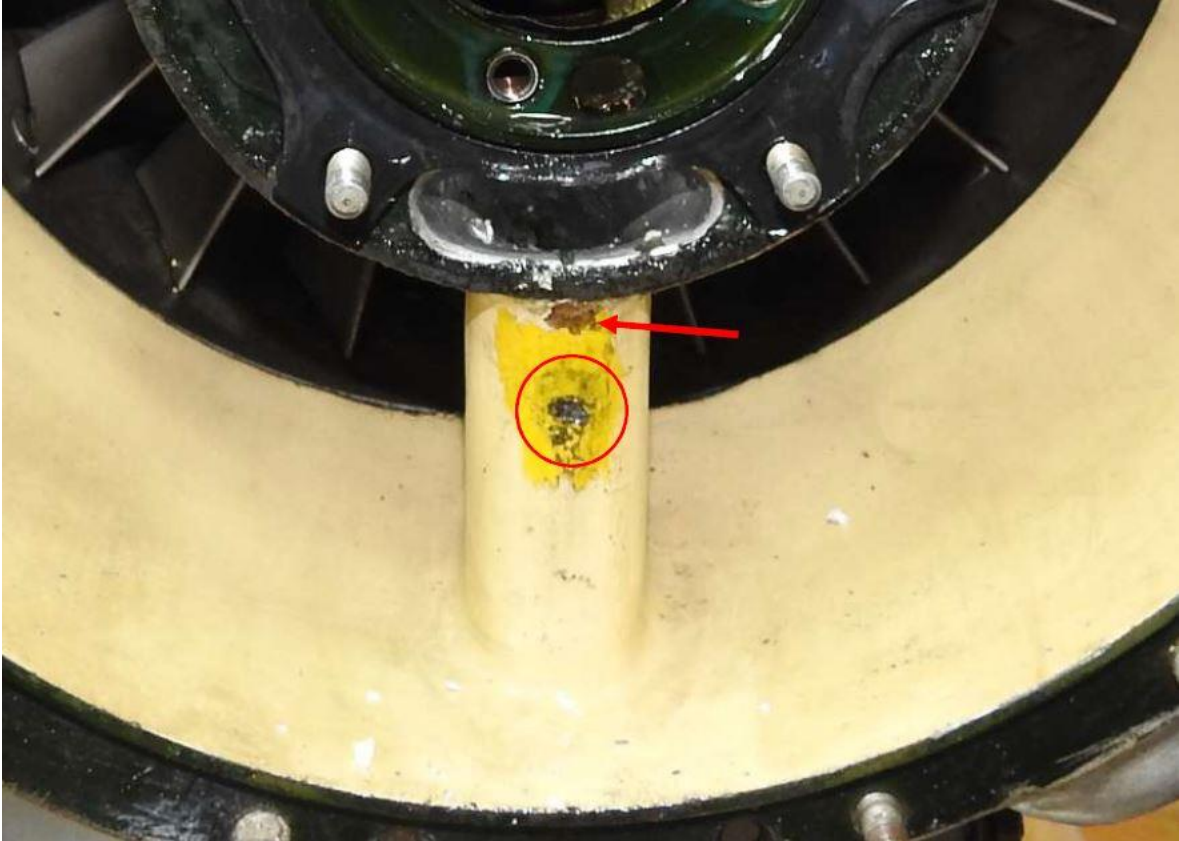
Figure 21: Corroded airflow ducts
