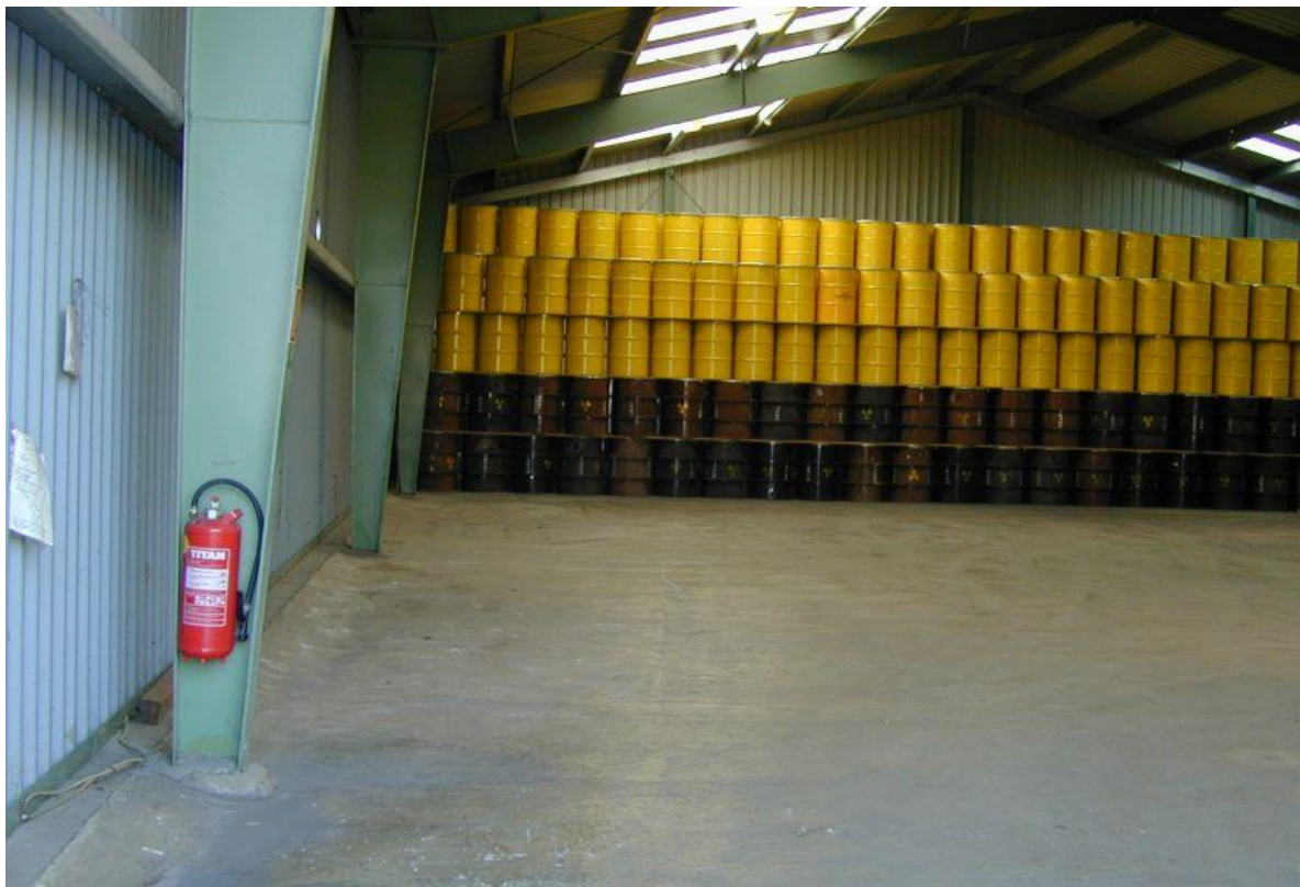
Figure 4 Conditioned waste in interim storage facility 12A, © NES
