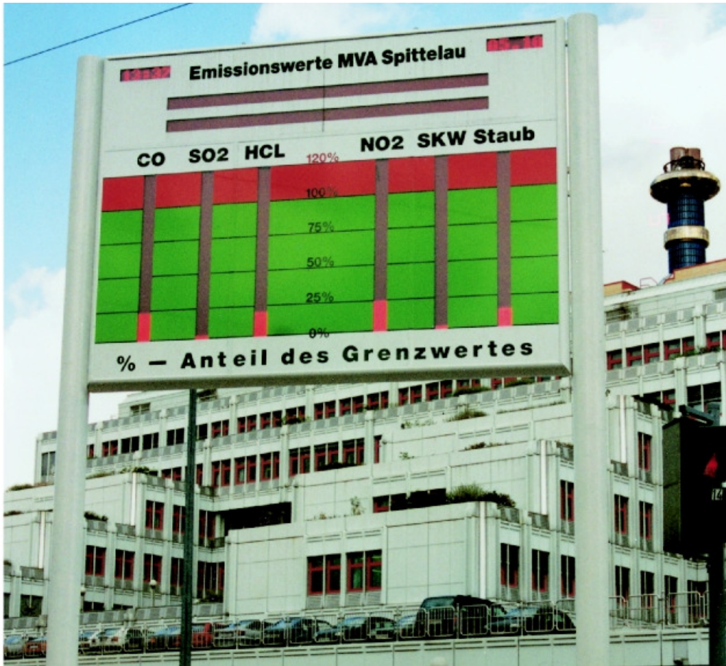
Public display panel with the current emission data of the waste incineration plant Spittelau in Vienna
