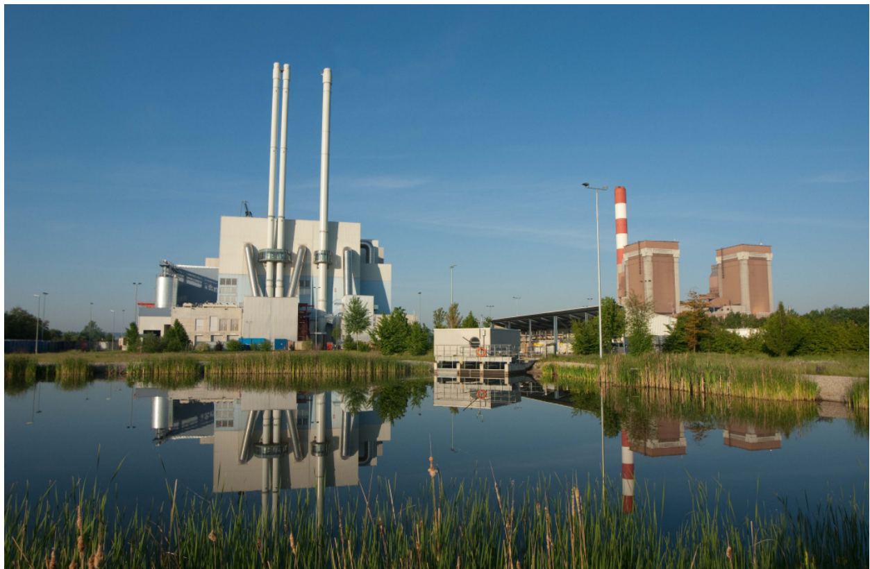
View of the EVN waste incineration plant linked to the neighboring coal-fired power plant Dürnrohr in Lower Austria
