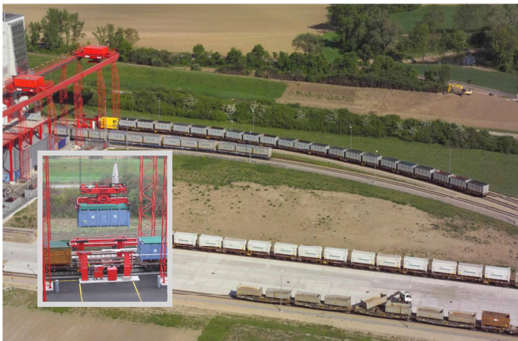
Unloading possibilities for waste shipped by train to EVN Abfallverwertung (automatic unloading of containers by crane or unloading by truck)
