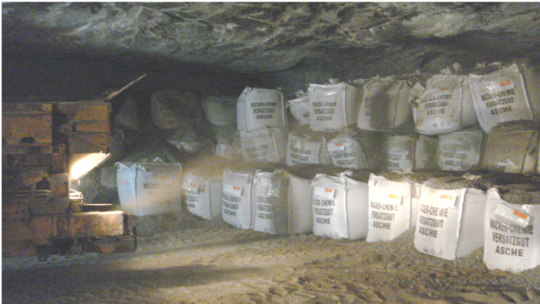
Example for the backfill of underground caverns in massive salt formation with inorganic hazardous waste material packed in big bags. The space to the ceiling is backfilled with “waste rock” from mining by a belt slinger machine.
