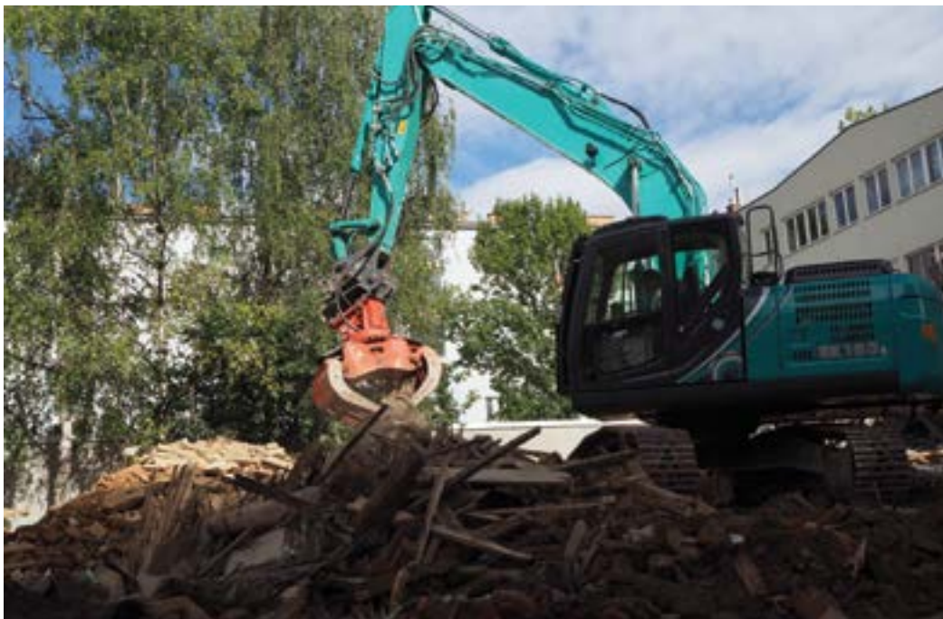
Figure 10: Demolition work is especially relevant with regard to waste.
