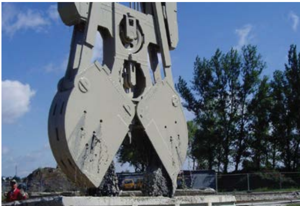
Figure 159: Slurry wall excavation
