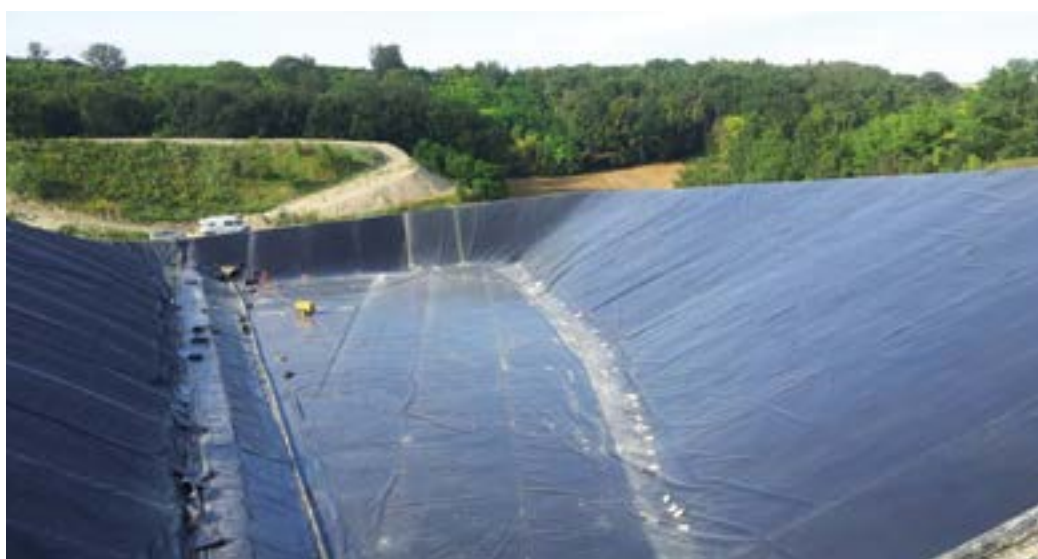
Figure 15: Landfill base sealing
