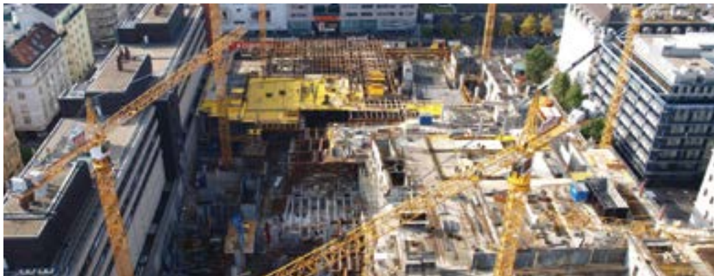
Figure 97: Building activities cause considerable waste quantities.
