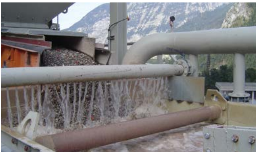
Figure 68: Wet processing of mineral construction and demolition waste
