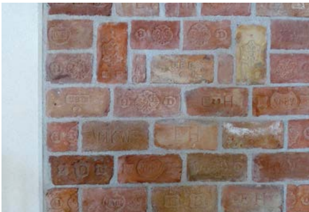
Figure 92: Reuse of building components
