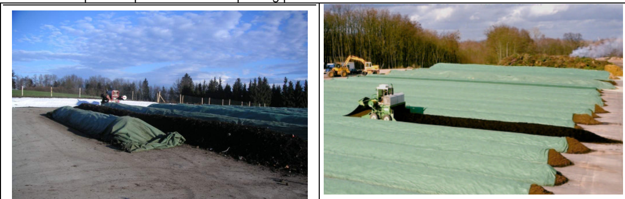
Fig. 6-3. Two examples of typical paved open windrow composting plants with one sided slope of ca. 5 %
