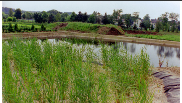
Fig. 6-7: biological water purification in reed grass beds and water retention basin
