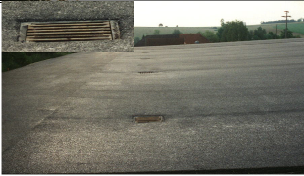
Fig. 6-6. Slope of sealed composting plant drains the water into a simple gully
