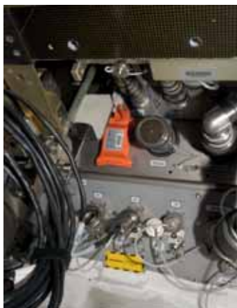
DOSIS badge installed in the Human Research Facility rack
